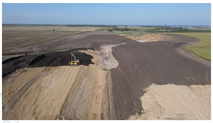
08/31/2023: Topsoil placement near structure C2 (Looking downstream)
